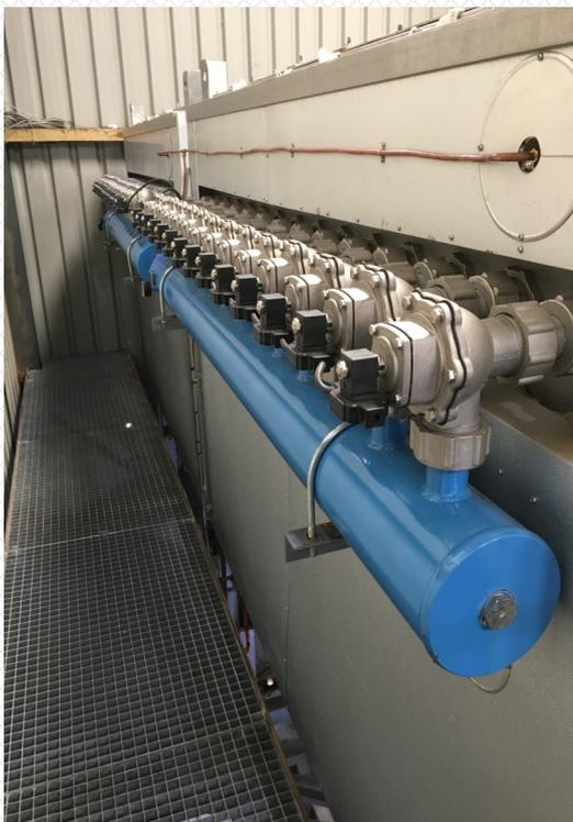
Site work was kept to the minimum by the filters arriving completely built, only needing to be lifted into position on top of their new support frames. Site electrics were completed within a day and the new duct work was erected by the site's maintenance fitters, again keeping costs to the customer down.
