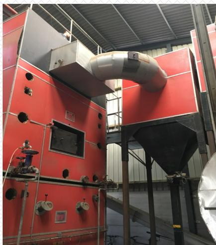
Space within the existing boiler house was limited, but by using a bespoke design it was possible to locate the filter adjacent to the boiler. This entailed raising the filter higher than normal off the ground above the existing ash conveyor.
